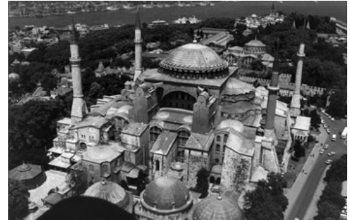
Cathedral of Hagia Sophia in Constantinople, site of the excommunication of 1054. The building today reflects recent additions of Islamic art and architecture.
