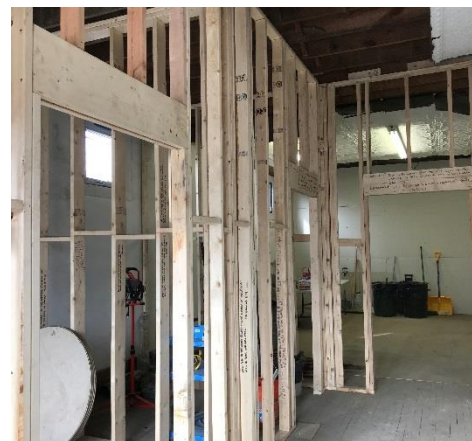
View - Bathroom into Kitchen
