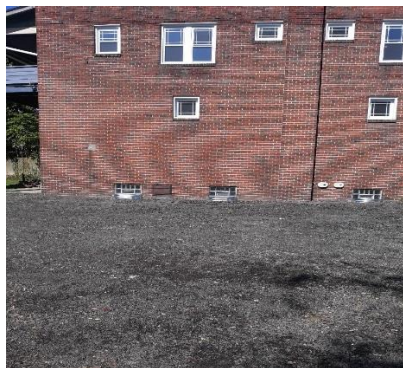
New Parking Lot
