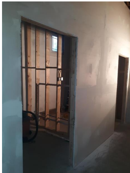
Bathroom framing and walls
