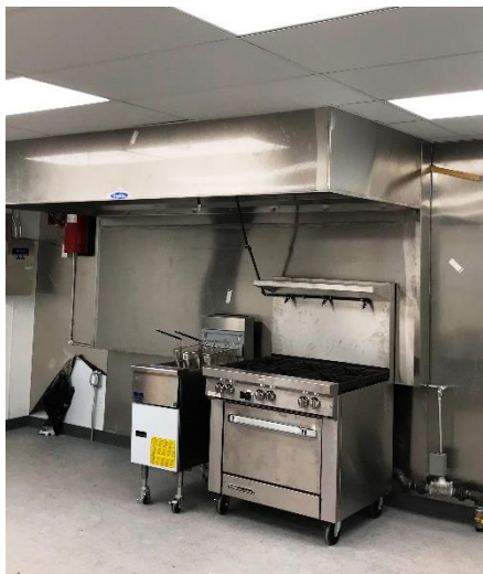
New Kitchen – almost complete!
